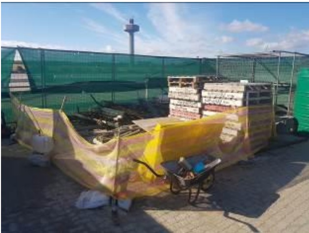
Image 4: Storage of materials within the site camp.
