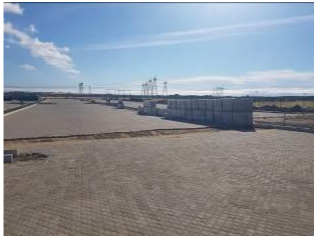
Image 5: Laid paving infrastructure.
