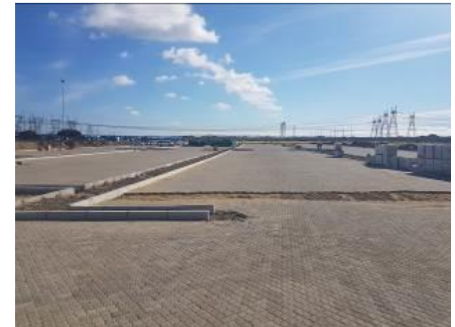
Image 6: Curb areas to be filled.
