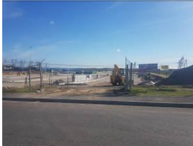
Image 2: Second access point to site, with site notices.
