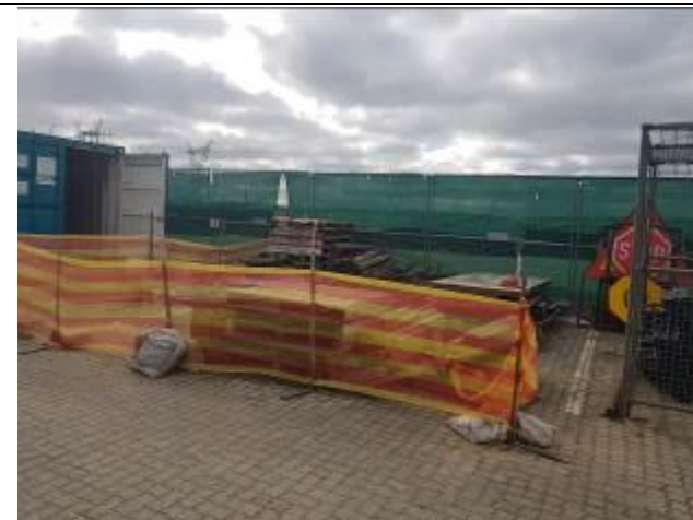
Image 14: Storage of construction materials within the site camp.
