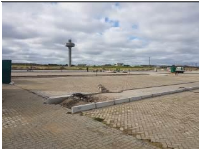
Image 12: Curb infrastrure backfilled with excavated material.
