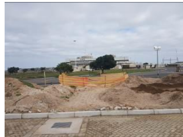
Image 17: Demarcation of excation.
