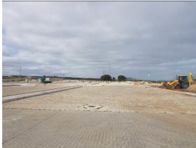
Image 10: Paving infrastructure in place.
